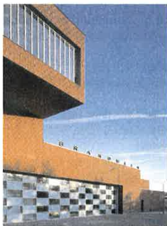
Brandweerkazerne, Breda Architect: Neutelings Riedijk
